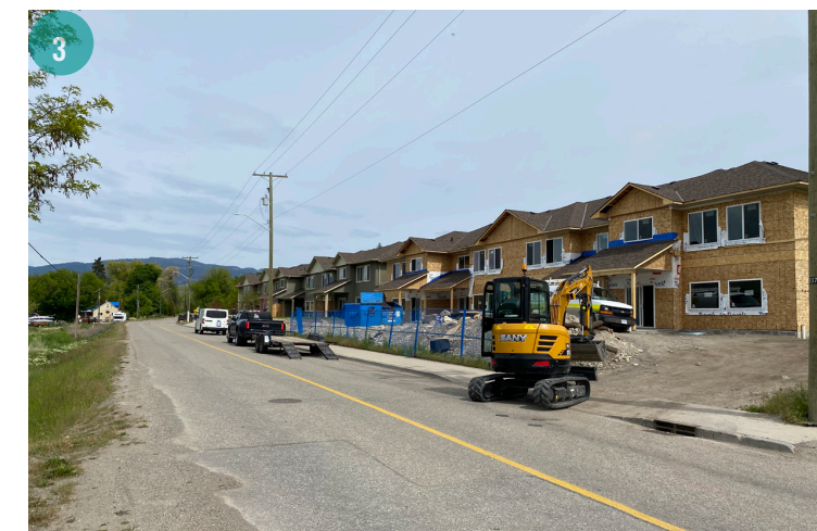
New Townhouses Under Construction
